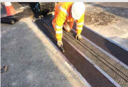
Image of T-Mat bridge expansion joint
